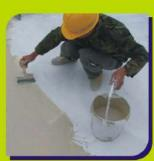
Multi Purpose Waterproofing Coating / Membrane
